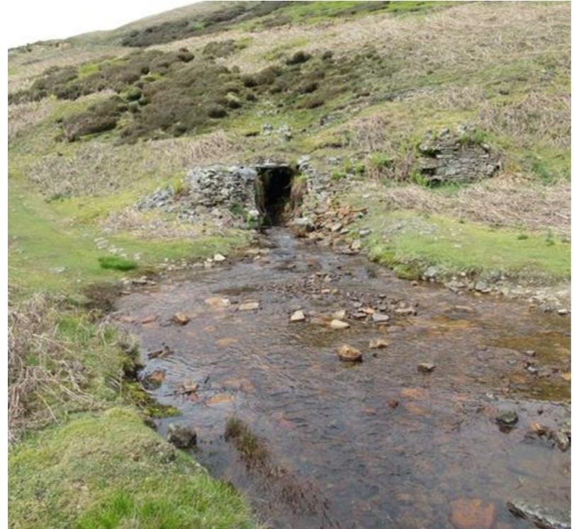
Old lead mining level and ford. © Copyright Les Hull
